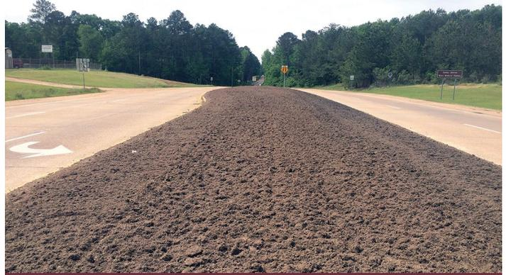
Figure 1. This elevated median was tilled before sowing. Multiple passes over a site may be required to break down large clods. A smooth soil surface prevents broadcast seed from getting buried too deep between clods during weathering.
