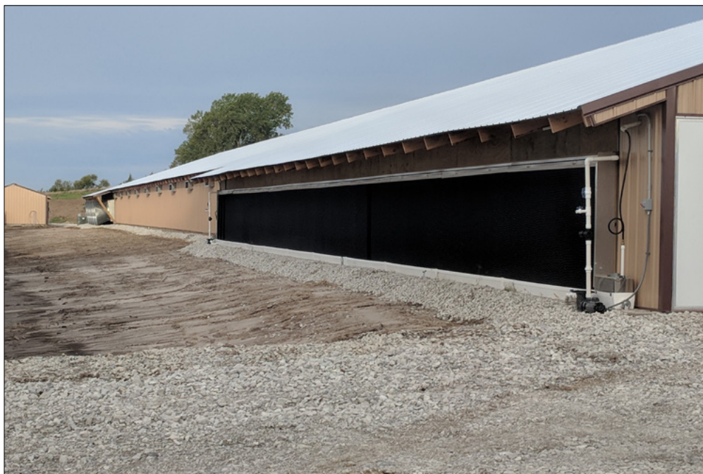
Figure 1. A typical broiler house with an evaporative cooling system and tunnel exhaust fans. The exhaust fans are visible at the far left, while the evaporative pads are in the foreground. This particular system has two pumps on either end of the pads supplying water toward the center.
