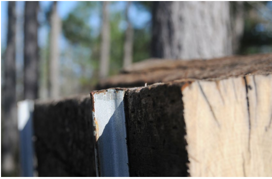
Figure 3. The T-posts should be level with the back of the top layer of cross ties once the structure has been constructed. This is to prevent any ricochet from a projectile striking the metal of the T-post.
