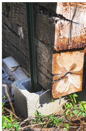
Figure 2. Next, drive the T-posts into the back left and right cinder blocks. These T-posts provide support for the cross ties as they are stacked.
