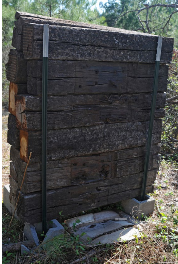
Figure 5. Once completed, the backstop should not be leaning or unstable.
