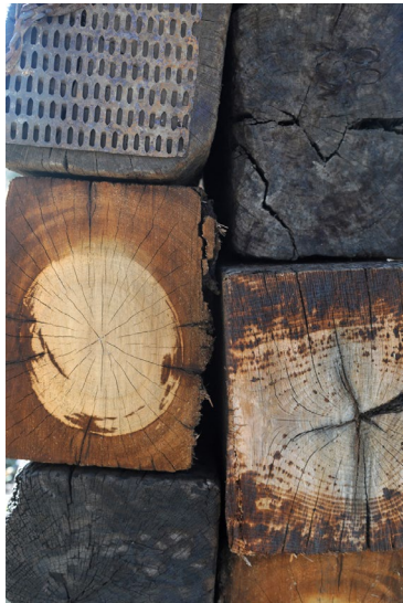
Figure 4. Cut the cross ties in half and stack them two deep with the long side facing out. As you are stacking the cross ties, make sure the seams of the back layer are offset from the front layer. This will prevent a projectile from passing through the backstop.
